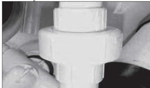
**Step 2:** Unscrew the fitting to expose the strainer.
