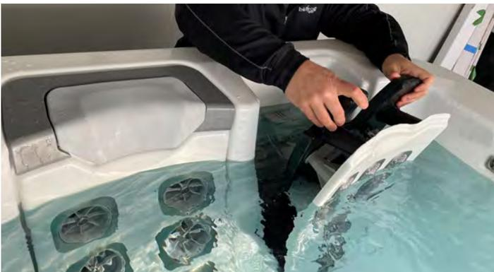
**Step 3:** Remove the Simplicity filter holder. Reach down into the jet pod and grab the handle, push toward the middle of the spa and lift up to remove from the housing. Place holder on a flat
